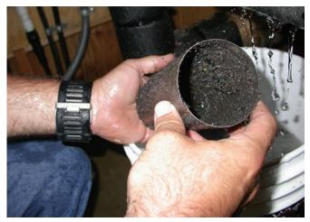
**Photo 1:** Ground loop and building systems must be properly flushed and purged of debris. Debris clogs system equipment and biological material contributes to a drop in water pH as it decays.
